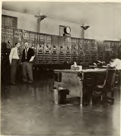
POWER FOREMAN, (standing right)
